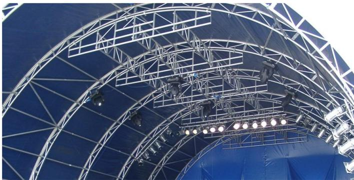
The 12.2m span Alidome can be supplied with an in-built lighting grid that is capable of supporting a lighting payload of up to 500kg per 2.44m deep bay.
